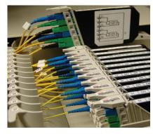
Splitters can be checked for damage by scanning in a method similar to that used for fiber bend and break testing. In addition, ports can be checked end on for the presence of light or by bending output fibers over a finger or mandrel. Splitters with division ratios as high as 1:32 are verifiable in this way due to the high sensitivity of the PX-Q500. WDM devices can also be tested with the use of narrow band heads to verify proper wavelength diversion.
