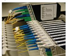
Splitters can be checked for damage by scanning in a method similar to that used for fiber bend and break testing. In addition, ports can be checked end on for the presence of light or by bending output fibers over a finger or mandrel. Splitters with division ratios as high as 1:32 are verifiable in this way due to the high sensitivity of the PX-Q550. WDM devices can also be tested with the use of narrow band heads to verify proper wavelength diversion.
