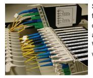
Splitters can be checked for damage by scanning in a method similar to that used for fiber bend and break testing. In addition, ports can be checked end on for the presence of light or by bending output fibers over a finger or mandrel. Splitters with division ratios as high as 1:32 are verifiable in this way due to the high sensitivity of the PX-Q650. WDM devices can also be tested with the use of narrow band heads to verify proper wavelength diversion.
