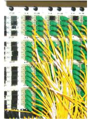
In situations where patch cords are connected to the output ports, simply bending patch cords over a finger will permit tracing. When used with Photonix high power tracer sources, the PX-Q650 can even trace ports through most plastic end caps or by connector bulkhead leakage.
